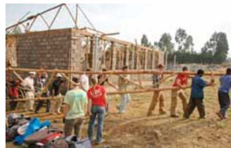
Building in Process – Addis Ababa, Ethiopia
