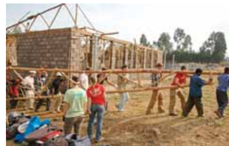
Building in Process – Addis Ababa, Ethiopia
